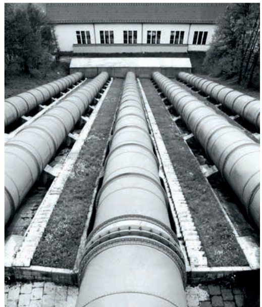
From the canal, the water flows through the pipes of the Alz power plant, then down to the Salzach River, which has its source in the Alps
