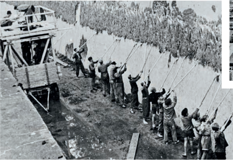
The canal is cleaned out every once in a while, formerly by manual labor (undated picture), now by machines
