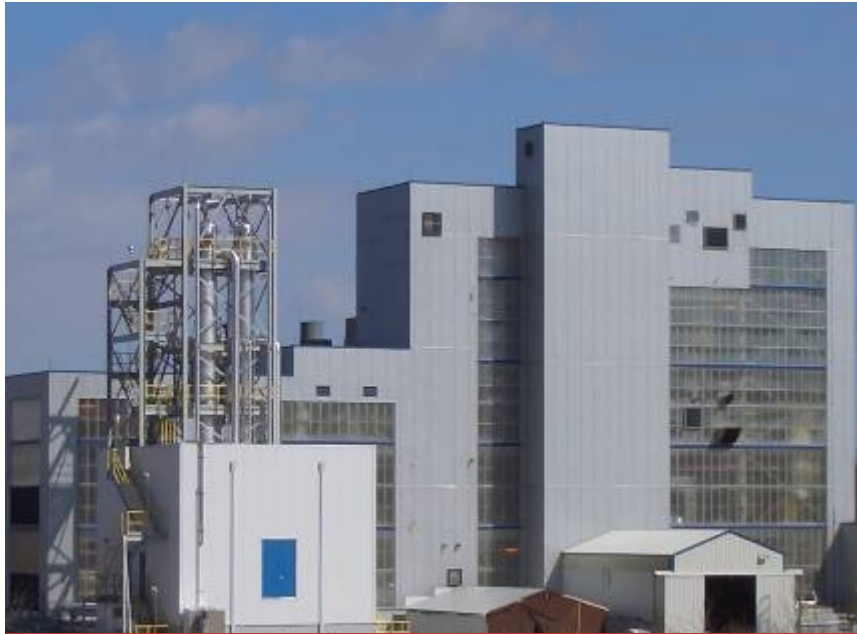
Production facility for cyclodextrins at Eddyville (USA)
