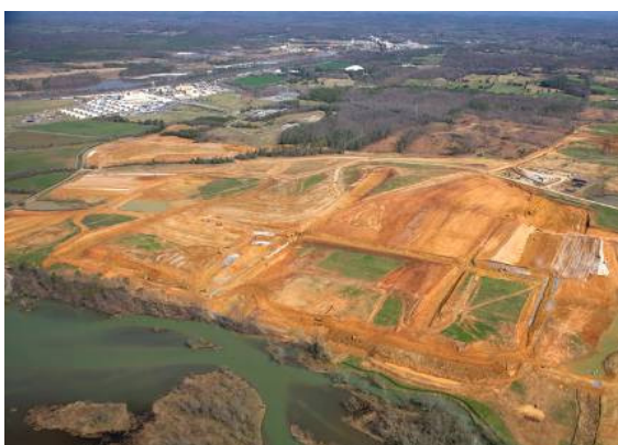
Aerial view of construction site
