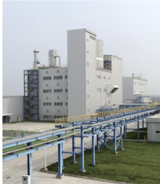
PVAc solid resins facility in Nanjing (China)
