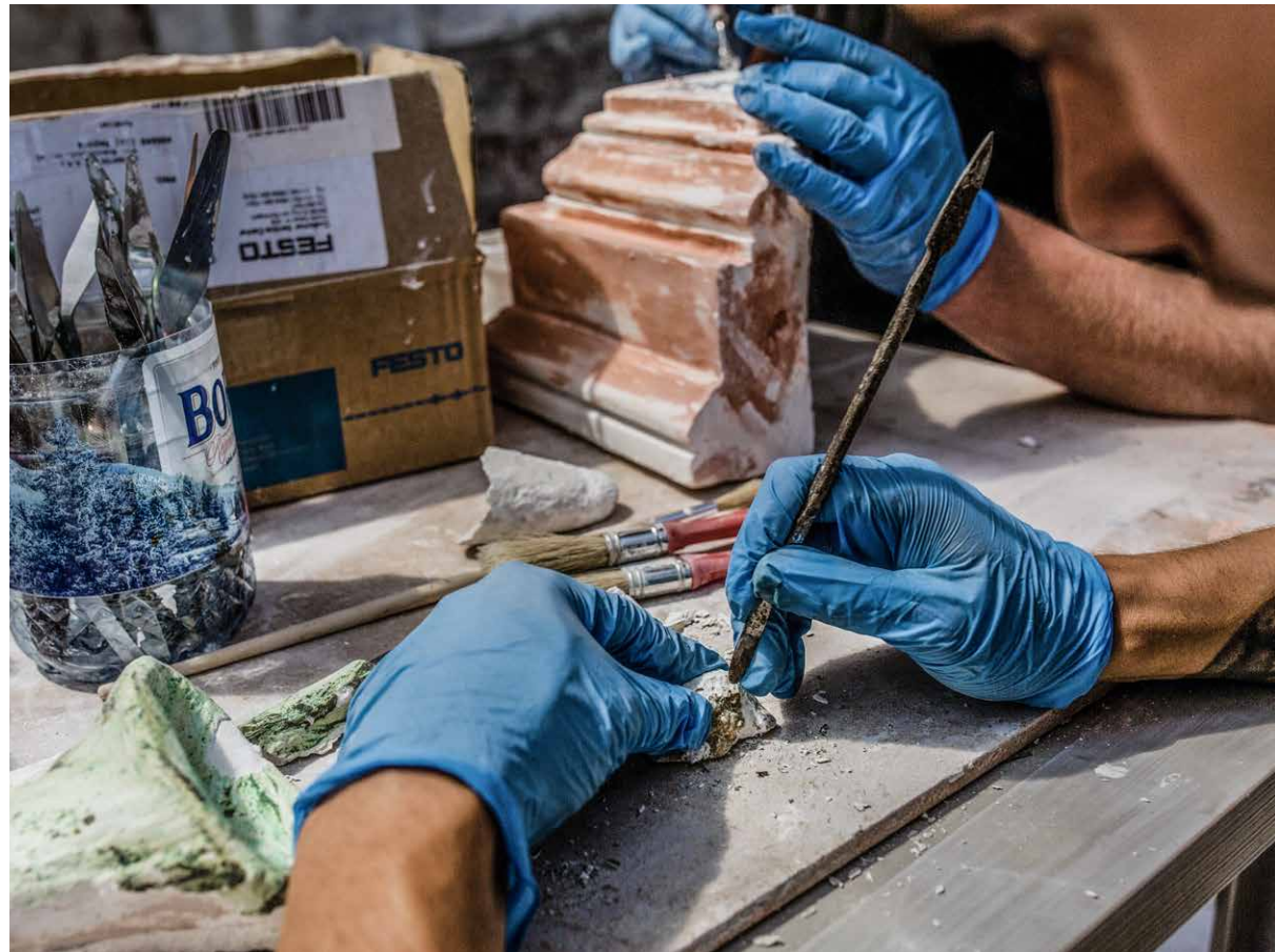
The restorers carefully remove the many layers of the past decades to reveal the original fabric of the building.
