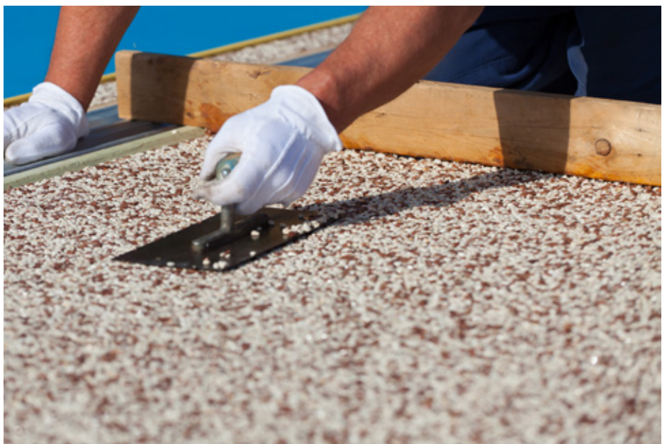
Stone carpet with typical particle size of 2–4 mm
