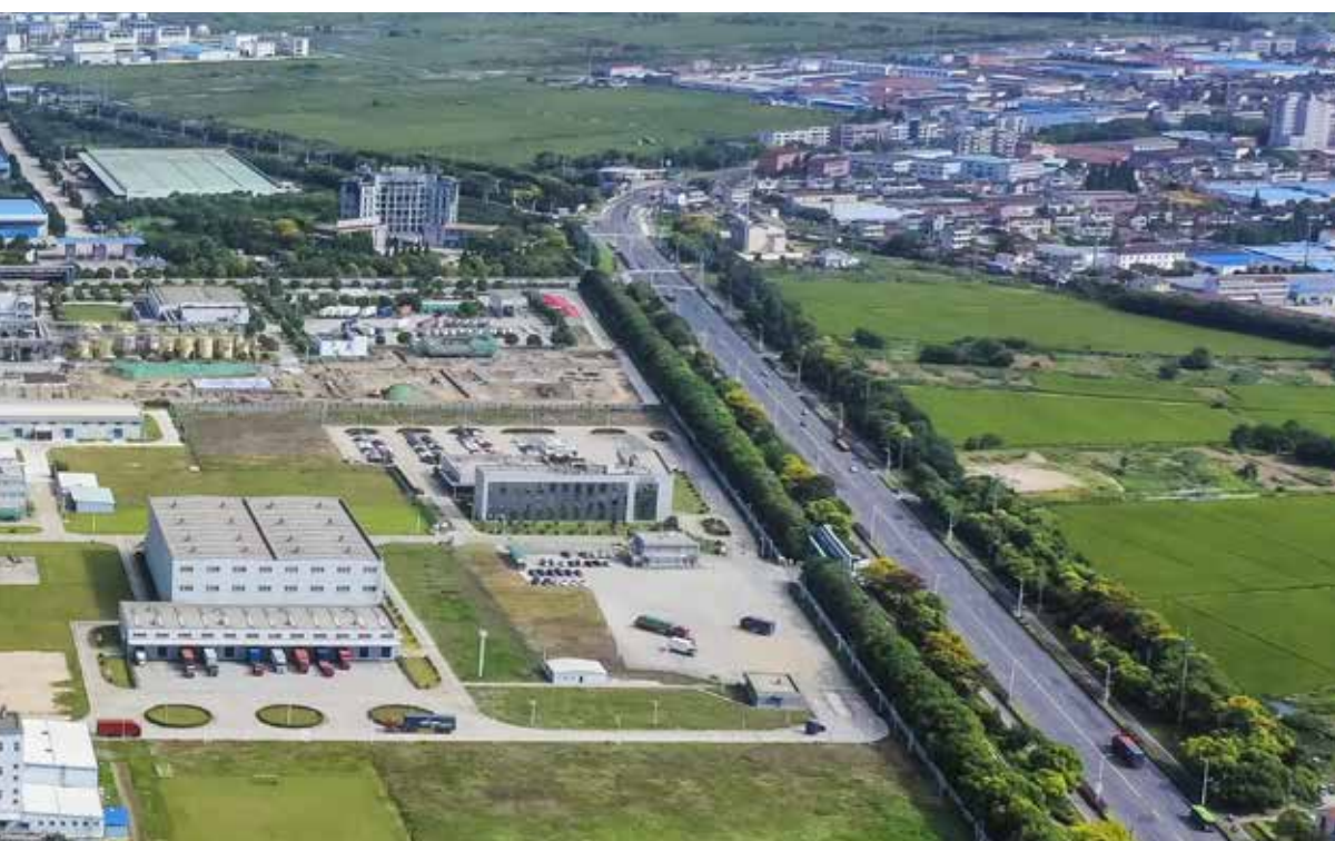
WACKER Zhangjiagang integrated silicone manufacturing site
