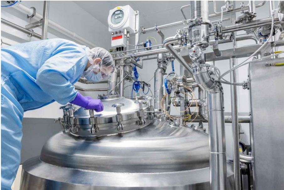
Lipids that are used to formulate mRNA active ingredients are stored in large steel tanks. (Photo: WACKER)
