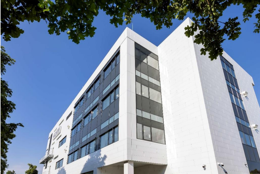
More than 100 highly qualified jobs have already been created for the mRNA competence center at WACKER's site in Halle. (Photo: WACKER).
