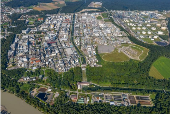
Caption: An aerial view of the Burghausen site. BARA can be seen in the lower part of the picture.
