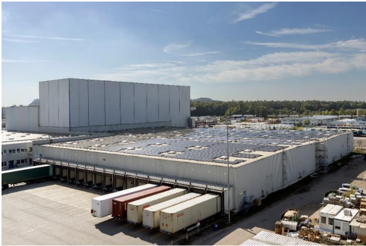
Caption: Photovoltaic systems were installed on several large sections of roof at the Burghausen site in 2023.
