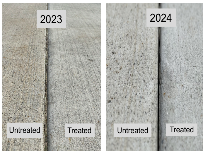
Figure 9. Poured (ready mix) in driveway at AIC with treated and untreated concrete slab poured in 2021 and then evaluated in 2023 (left) and 2024 (right).
