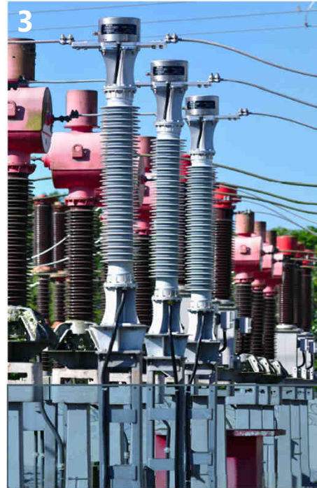
3 | Foam-filled CHSPs – 145 kV for optical CT
