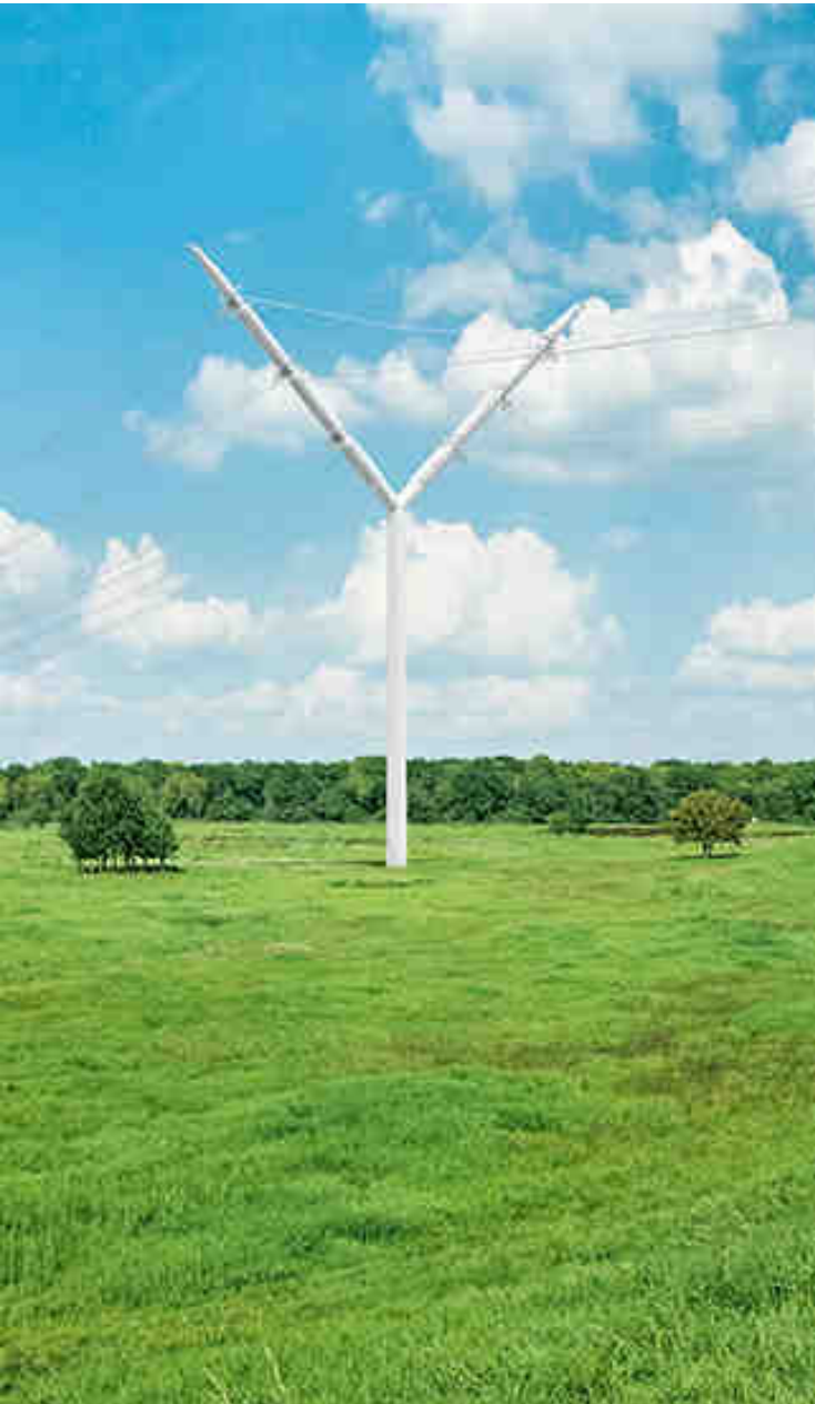
Demonstrator of 400 kV European Composite Pylon
