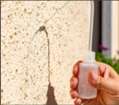
The water-beading test shows: Droplets simply roll off the walls – the coating is still watertight, even after 20 years.
