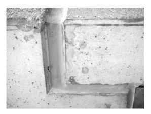
Metal, natural stone or concrete are substrate materials to which sealants often do not adhere properly. Joints should therefore be coated with a primer before the sealant is applied.
